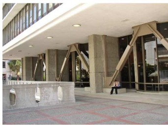
Buckling Restrained Brace
